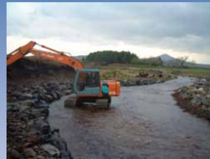
Rehabilitation work on the Srahnaploya River
